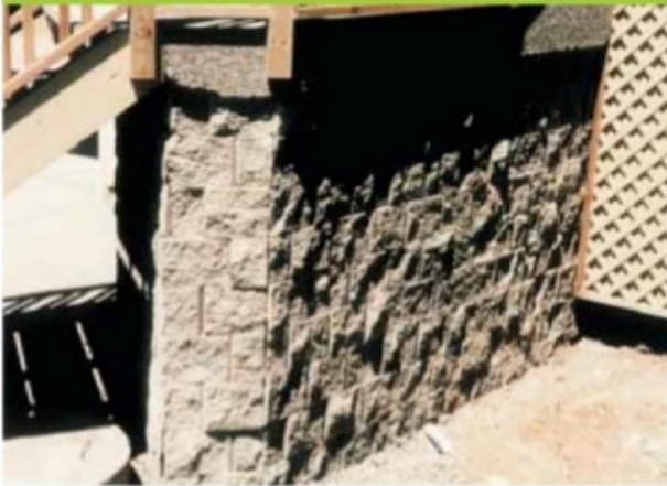
Two further examples of architectural features
