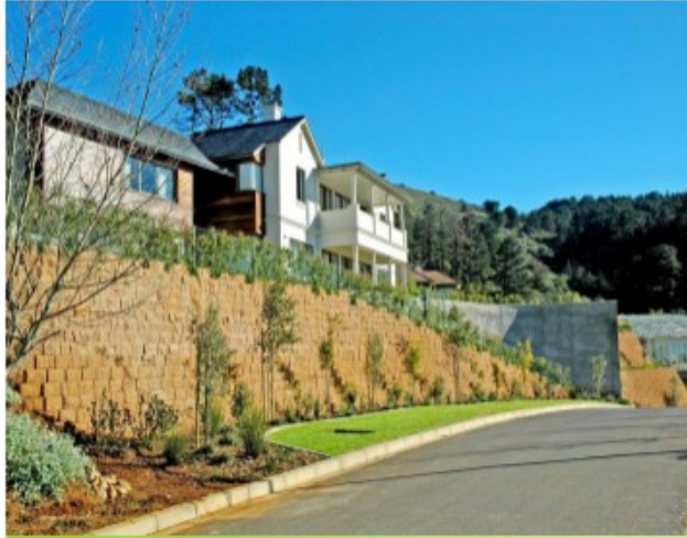
Retaining wall created with Rockface showing to create a garden.
