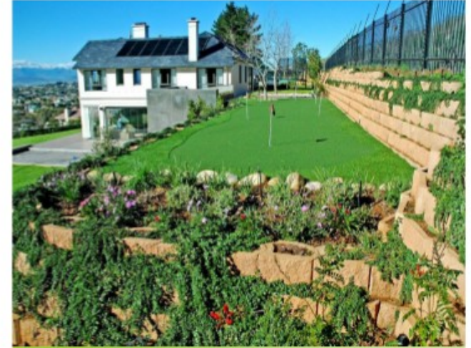
Practical retaining wall creating functional areas with no compromise on design.
