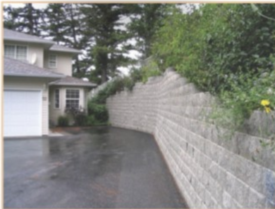
NEAR VERTICAL, COMPOSITE WALLS
