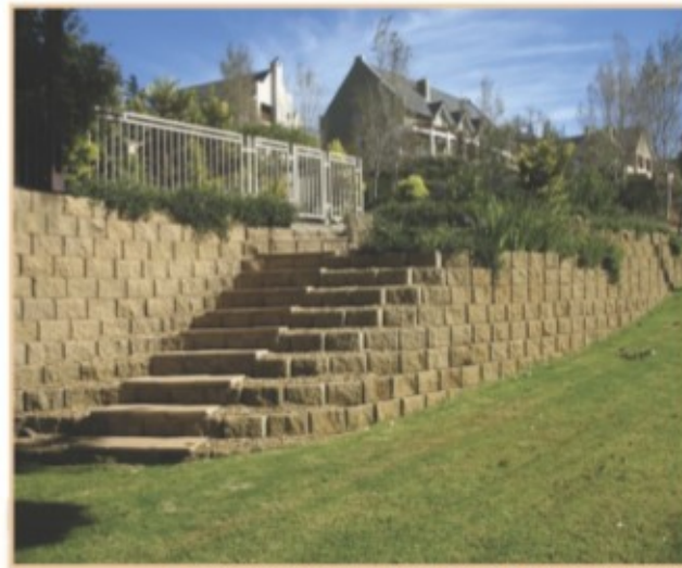
COMPOSITE WALLS IN SPLITFACE FINISH
